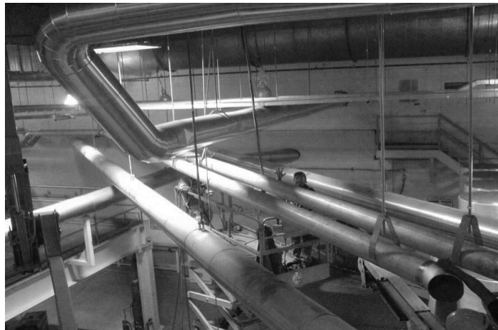
Figure 20: Pipe Installation at Machine Area
