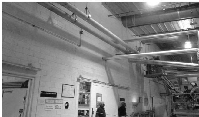
Figure 22: Working at Elevated Height
