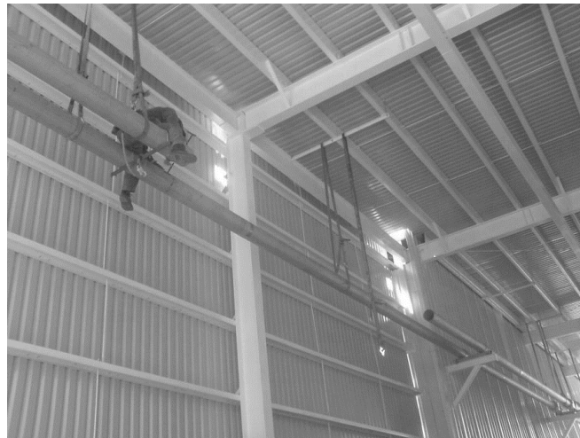
Figure 19: Pipe Installation at Railcar Area
