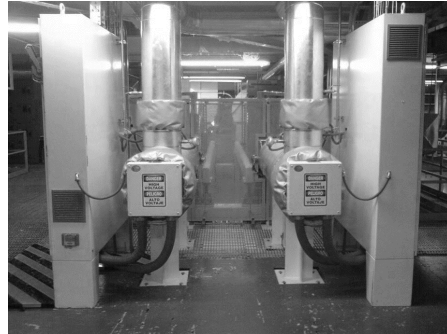
Figure 25: Installation of Air Heaters
