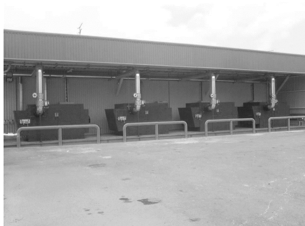
Figure 24: Finished Compressors Area
